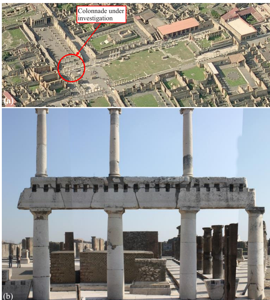
Figure 1: (a) The Forum in Pompeii: (a) Aerial view of the southern part of the Forum showing the colonnade under investigation, denoted with a red circle; (b) two-storey colonnade with multi-drum columns and multi-blocks segmented trabeation.
